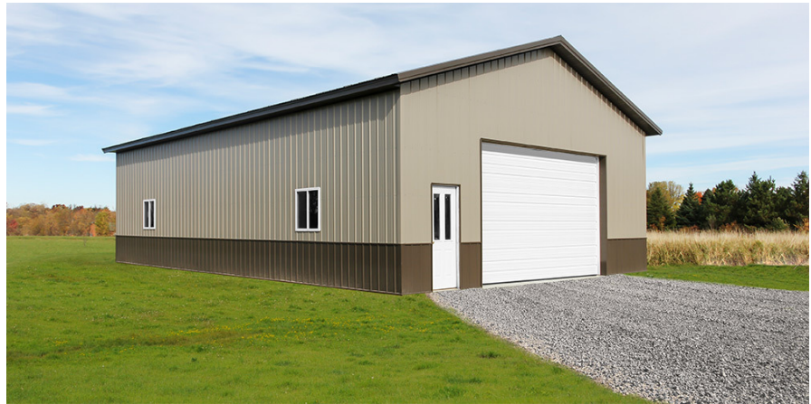
HB 2611 allows non-farm uses to occur in ag buildings that are exempt from the commercial building code
