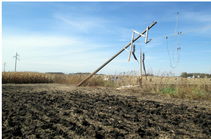
HB 2654 allows for better broadband access to rural Oregon without increasing conflicts with adjacent property uses
